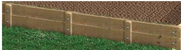
Sides secured by stakes
